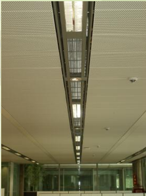
Chilled beams Air-Conditioning
